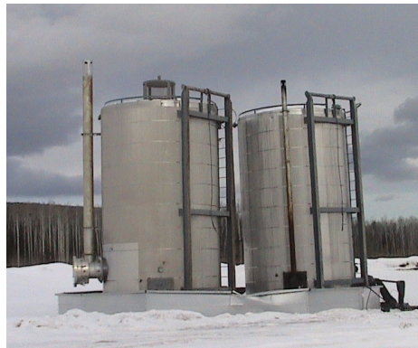
Figure 2: Environmentally friendly boiler system that reduces water disposal costs.
