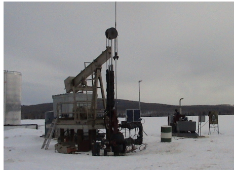
Figure 1: Vertical Hydraulic Pump on b-092.
