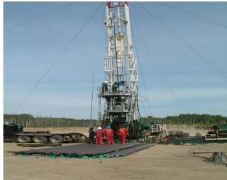
Figure 2: b-003-I Service Rig
